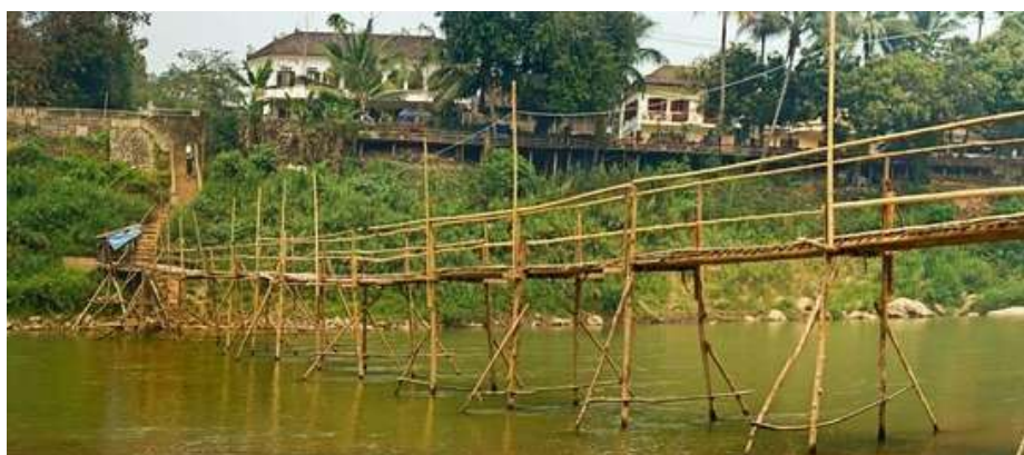
Figure 1: Example of a Pedestrian Bamboo Bridge in a typical Igbo indigenous community Photo credit: https://media-cdn.tripadvisor.com/media/photo-s/05/b5/d2/e5/bamboo-bridge.jpg
