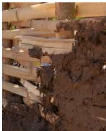
Figure 2: Bamboo split used as a skeleton wall prior to mud plastering
